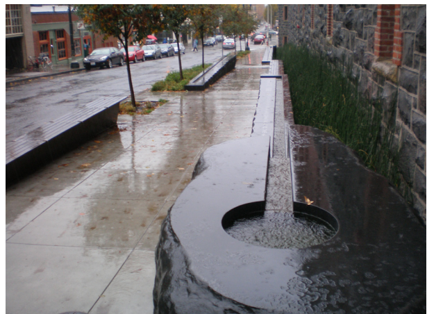
Stormwater runnels in Vera Katz Park in Portland, OR
