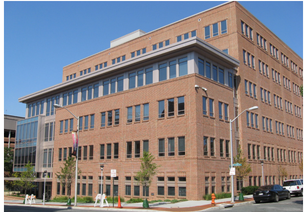
The Lexington Street Administrative Building creates a strong edge along both Lexington and Pearl Streets; it is also an example of a well-designed vertical setback.
