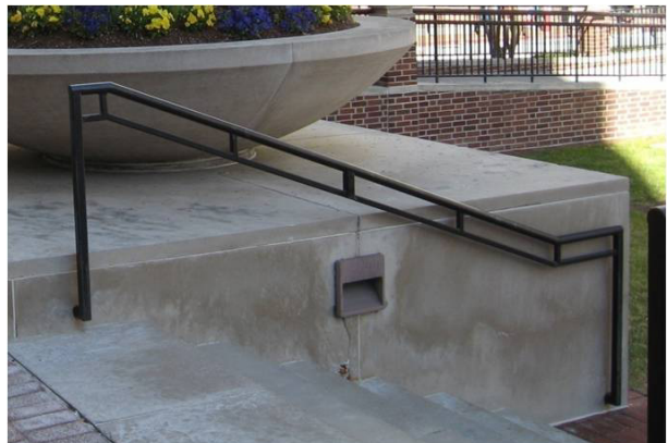
Handrail example on campus
