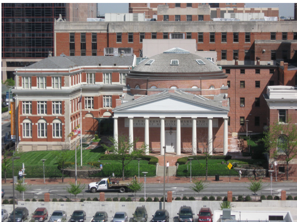
Historic Davidge Hall fronting Lombard Street
