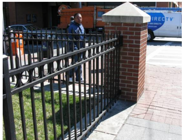
Example of existing secondary portal elements
