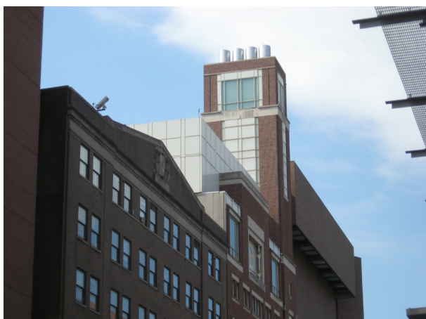
Across campus, roof styles span a century's worth of architectural styles.
