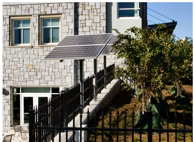
Solar panels at Emory University
