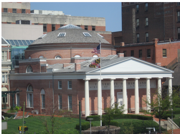
Classic Revival architecture of UMB's Davidge Hall
